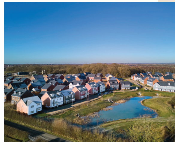
SuDS at Sevington Lakes, Ashford creates an attractive vista while mitigating flood risk across the development.
